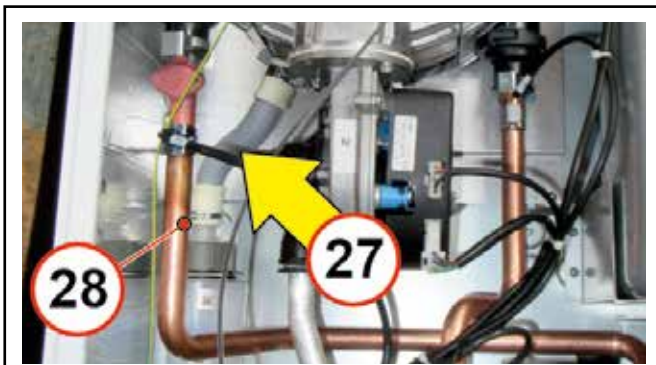
Connect corrugated tube (27) on the siphon, using spring 28 (as indicated).
